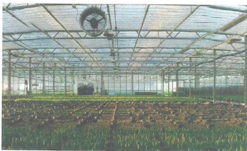
The dehumidifier saves the Swedish tulip and pot plant grower more than 60% on his total energy consumption because he can keep the screen and windows closed.
