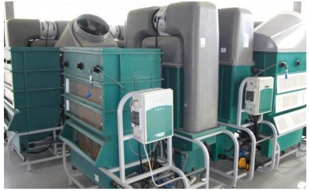
17 Eco Climate Converters are operating in the Netherlands and Germany. By drawing humid greenhouse air through a shower of salt, warm air is produced that can be used to heat the greenhouse. A beneficial side effect of this process is pathogenic fungi, including Botrytis and mildew, are killed. This helps to decrease the disease burden on greenhouse plants.
