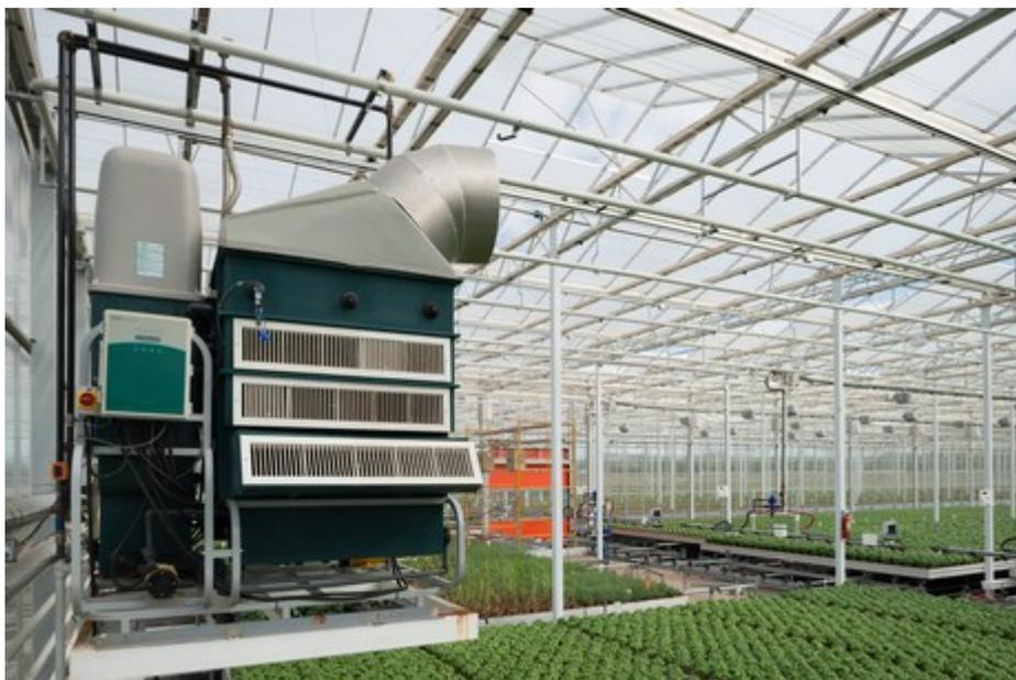
The Agam Ventilated Latent Heat Converter was developed to provide an alternative dehumidification strategy that at the same time would lower the disease pressure risk in controlled environments.
